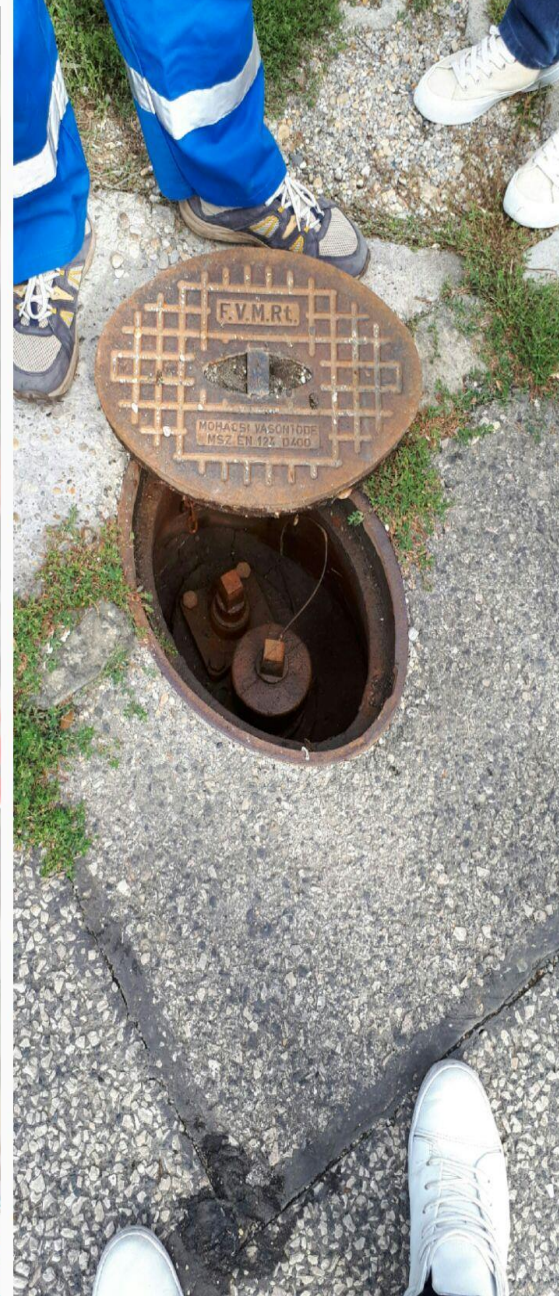
01417 – leaking hydrant
