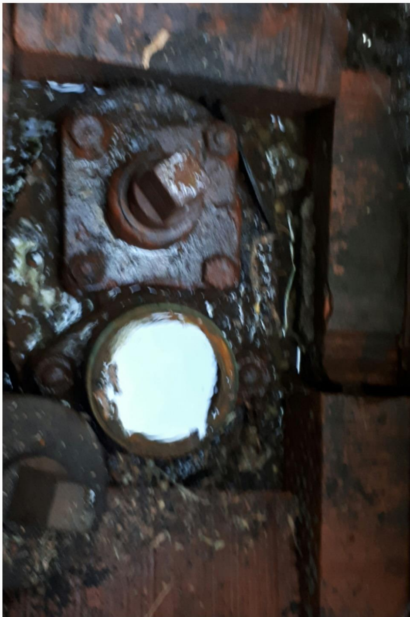
01452 – leaking hydrant valve
