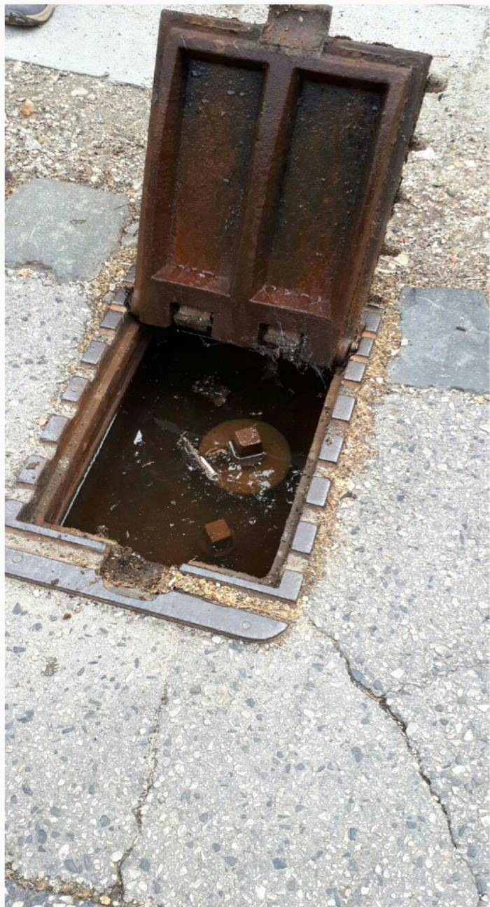
01416 – leaking hydrant
